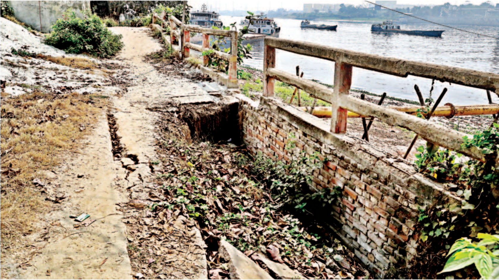
Neglect in maintenance has led to the collapse of a portion of the Buriganga riverside walkway at Kadamtali in Pagla, Narayanganj. Berthing of cargo vessels for unloading sand and bricks in the area also contributes to the damage. The photo was taken recently.
