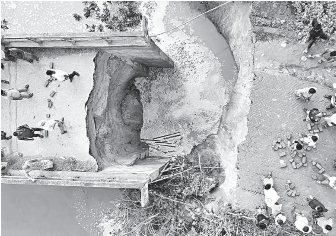
A large gap has appeared between the bridge and its approach road over the Dhaleshwari River in Tangail's Charabari area, cutting off communication with five surrounding unions after the west-side approach collapsed under heavy water pressure early yesterday.
