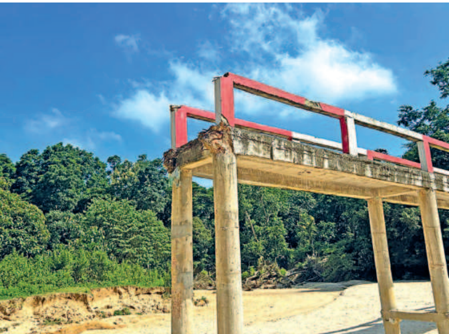
A partially collapsed concrete bridge in Tripura Palli, Chunarughat upazila, Habiganj. Local residents blame years of unregulated sand extraction from nearby hills for worsening erosion.
