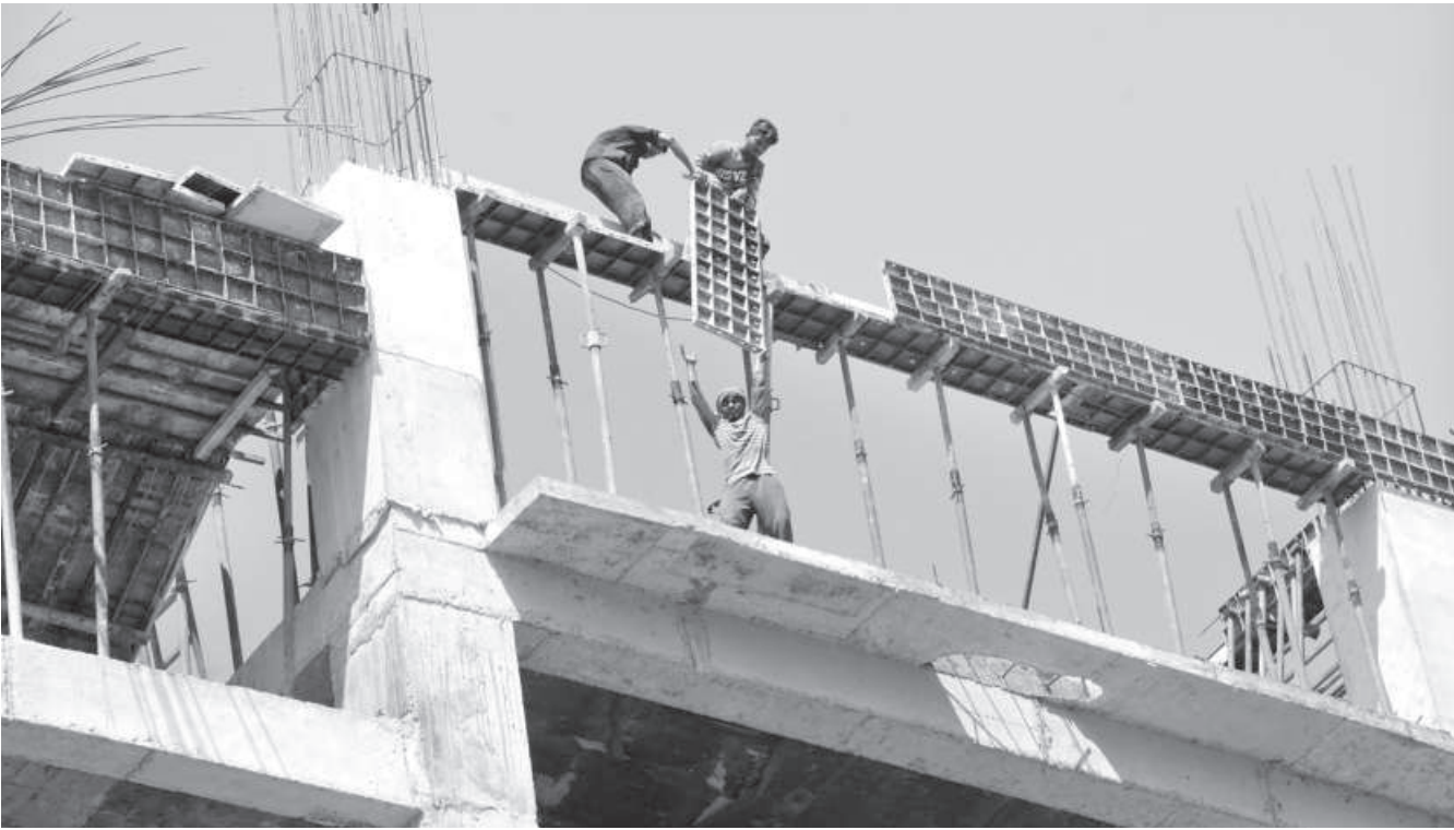
Workers at the Rajshahi University of Engineering and Technology construction site carry out their tasks without any safety equipment, exposing themselves to serious risks. A minor slip or error on this multi-story building could have fatal consequences.
