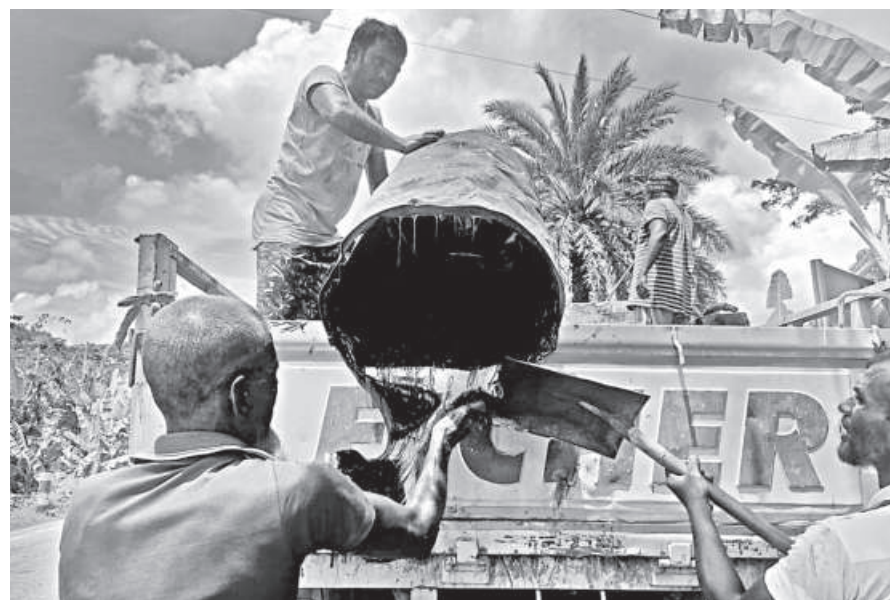
Workers of the Roads and Highways Department repairing a section of the Barishal-Dhaka highway, which was badly damaged by heavy rainfall. They are filling potholes with stone, sand, and bitumen to ensure the road is safe for vehicles. Working from morning to evening, each worker earns a daily wage of Tk 800. The photo was taken yesterday.
