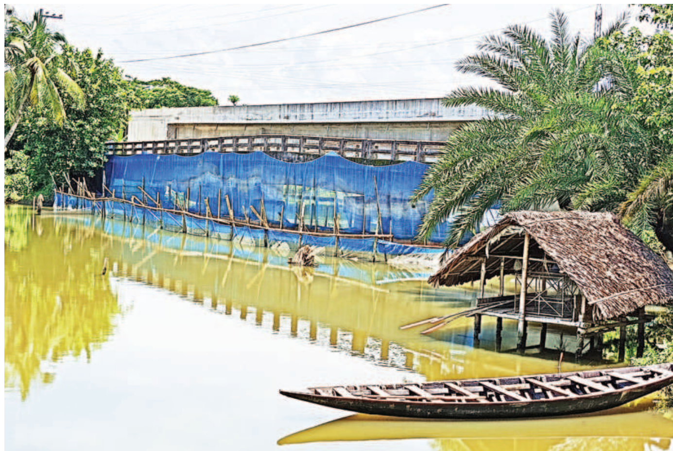
A cross-dam of nets and bamboo under Khegoraghat Bridge in Kashimpur village, Bagerhat Sadar, has blocked the Huji River's natural flow. Once vital for boats, fishing, and irrigation, the river is now largely divided into similar private fish enclosures. Photo was taken recently.
