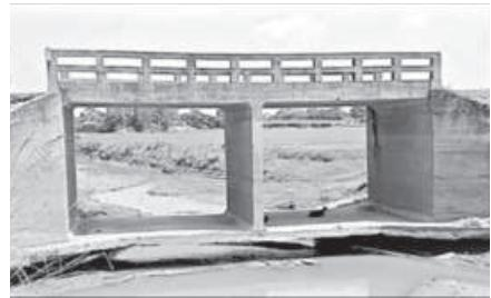
than before, eroding the soil beneath the bridge's pillars and deck. The bridge gradually lost ground support," said the PIO.
