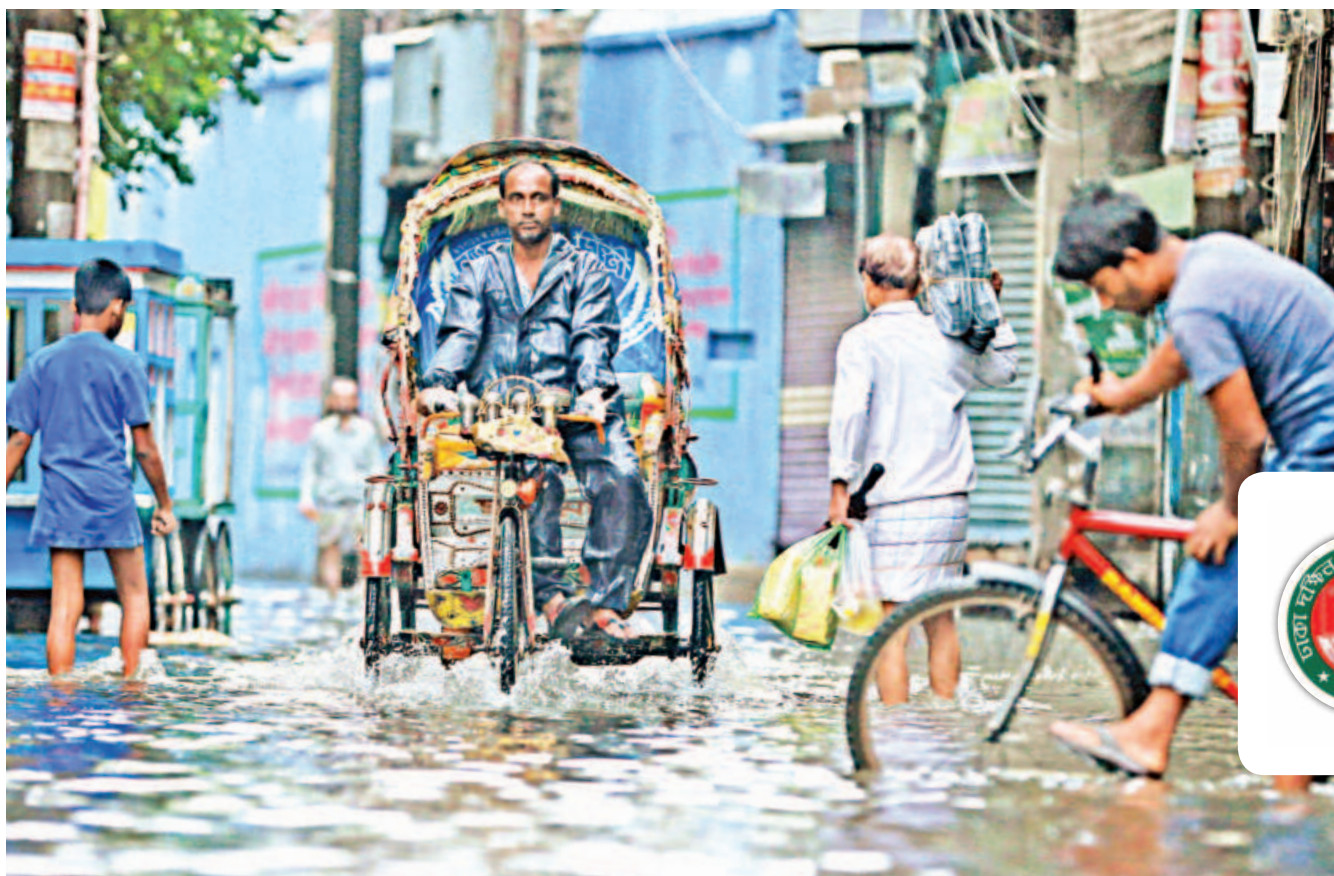
Even light rain causes significant waterlogging on this road in the Hussaini Dalan area of Old Dhaka, thanks to the absence of an effective drainage system. The photo was taken last week.
