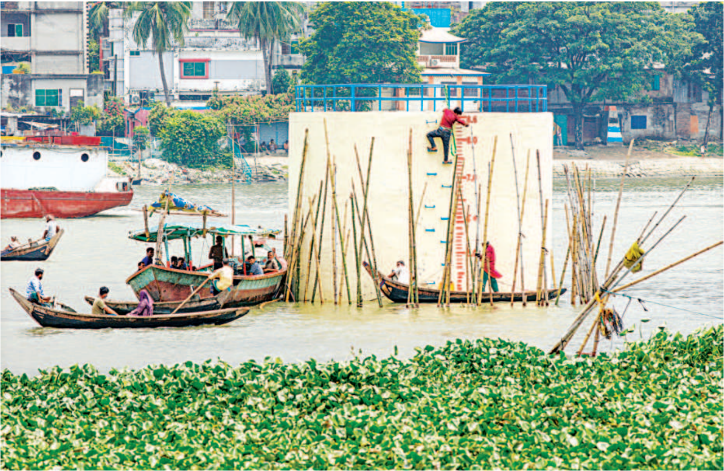
Bangladesh Inland Water Transport Authority workers measure the depth of the Buriganga to determine if any measures have to be taken to maintain the ideal level of water in the river. The structure has been in place for decades to check the water level at this point. The photo was taken from near the Kamrangirchar area of the capital yesterday.
