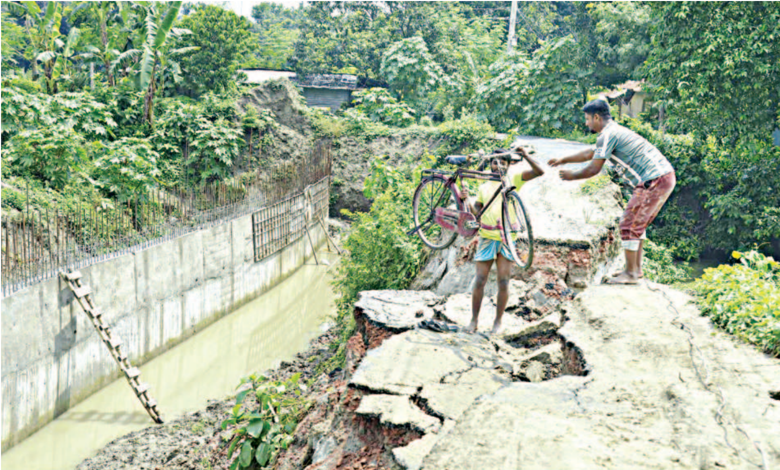
A man hands a bicycle to another across a broken stretch of the road from Pakuria Uttarpara to City Bypass in Rajshahi’s Paba, where large portions have collapsed. Locals say the contractor took no measures to protect the road during the construction of a wall beside it. The photo was taken yesterday.
