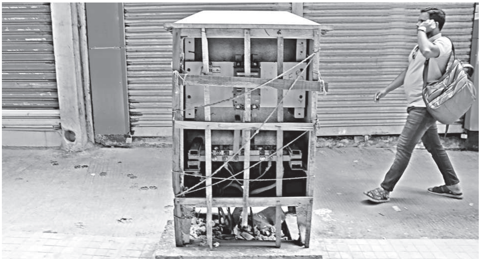
This high-voltage power box, connected to underground electrical lines, has been left exposed after its cover was broken. Nearby residents have used wood to create a temporary cover; however, it still poses a risk to passersby and anyone who comes into contact with it. Locals have alleged that, despite informing the authorities, no action has been taken to cover the exposed box. The photo was taken from Kazi Nazrul Islam Avenue, near the west side of the metro rail station yesterday.
