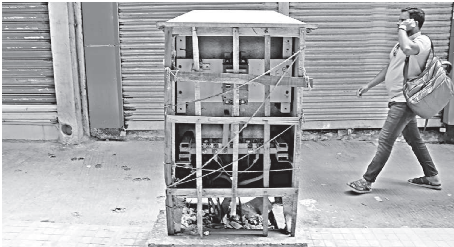
This high-voltage power box, connected to underground electrical lines, has been left exposed after its cover was broken. Nearby residents have used wood to create a temporary cover; however, it still poses a risk to passersby and anyone who comes into contact with it. Locals have alleged that, despite informing the authorities, no action has been taken to cover the exposed box. The photo was taken from Kazi Nazrul Islam Avenue, near the west side of the metro rail station yesterday.
