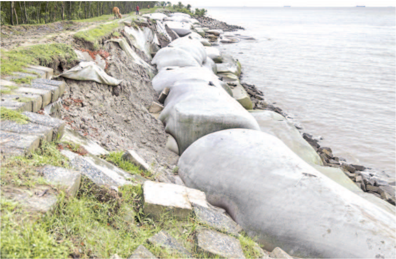
Cracks have appeared in the Tk 300-crore embankment in Chattogram's Banshkali upazila, just three years after its construction was completed in June 2022. Efforts to patch the damaged portions with sand-filled geo bags have so far proven ineffective, sparking fears of erosion among locals.
