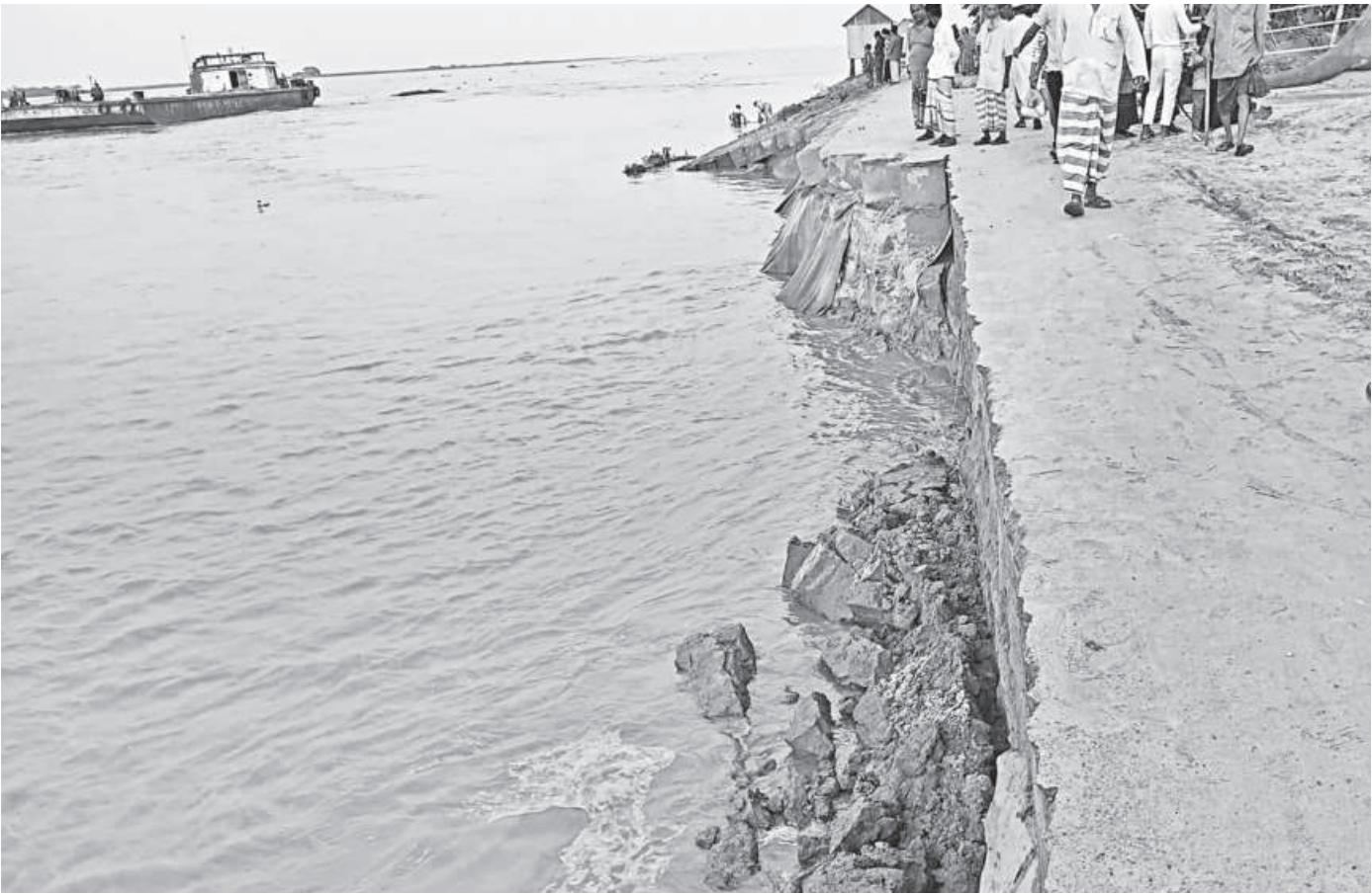
About 200 metres of the protective embankment near Naodoba Zero Point on the Padma Bridge in the Majhi Kandi area of Shariatpur collapsed into the river on Saturday morning due to erosion. Fearing further damage, three nearby shops were relocated. The photo was taken recently.
