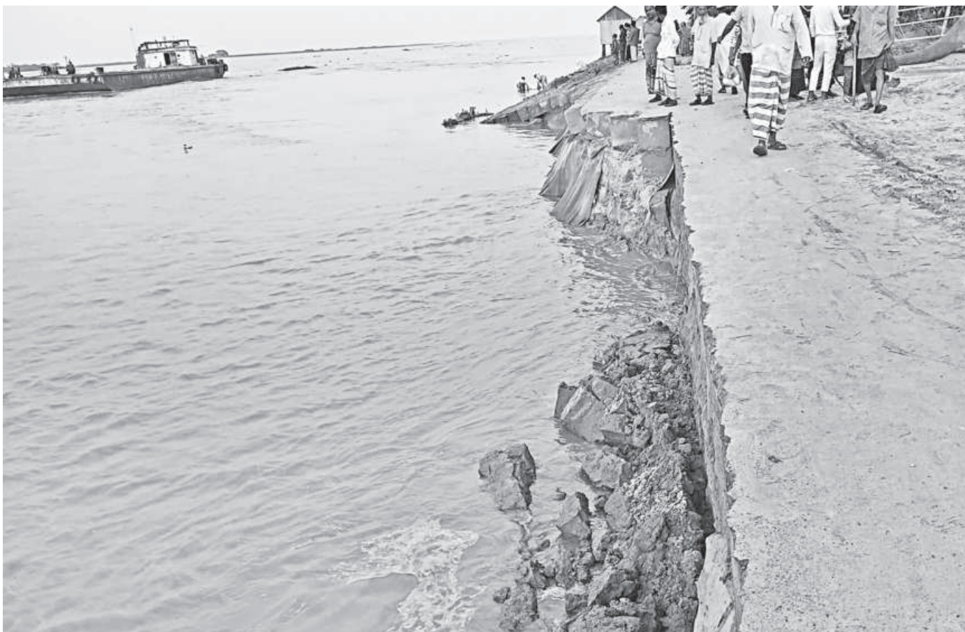
About 200 metres of the protective embankment near Naodoba Zero Point on the Padma Bridge in the Majhi Kandi area of Shariatpur collapsed into the river on Saturday morning due to erosion. Fearing further damage, three nearby shops were relocated. The photo was taken recently.
