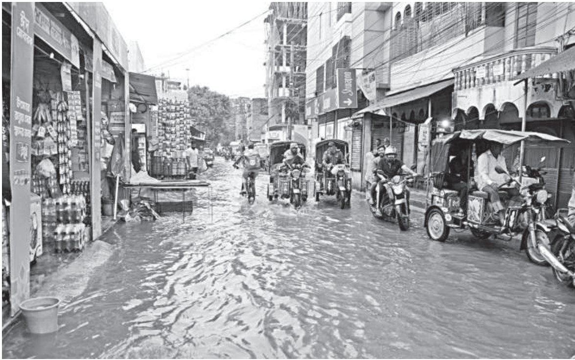
Just one hour of rainfall left this area in Rajshahi city waterlogged, with water entering alleyways and residential buildings. Locals alleged that poor drainage system was the major cause for constant waterlogging woes. The photo was taken from Baharpur area yesterday.
