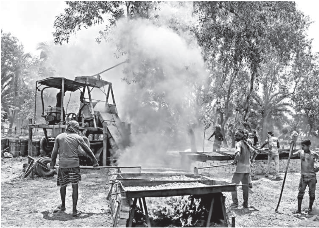
Black smoke covers the Rajbandh area of Khulna's Batiaghata as road repair activities continue using two burners to heat stones, which are then mixed with bitumen. The uncontrolled emissions from the burners and mixing machines are not only polluting the environment but also harming the local vegetation.
