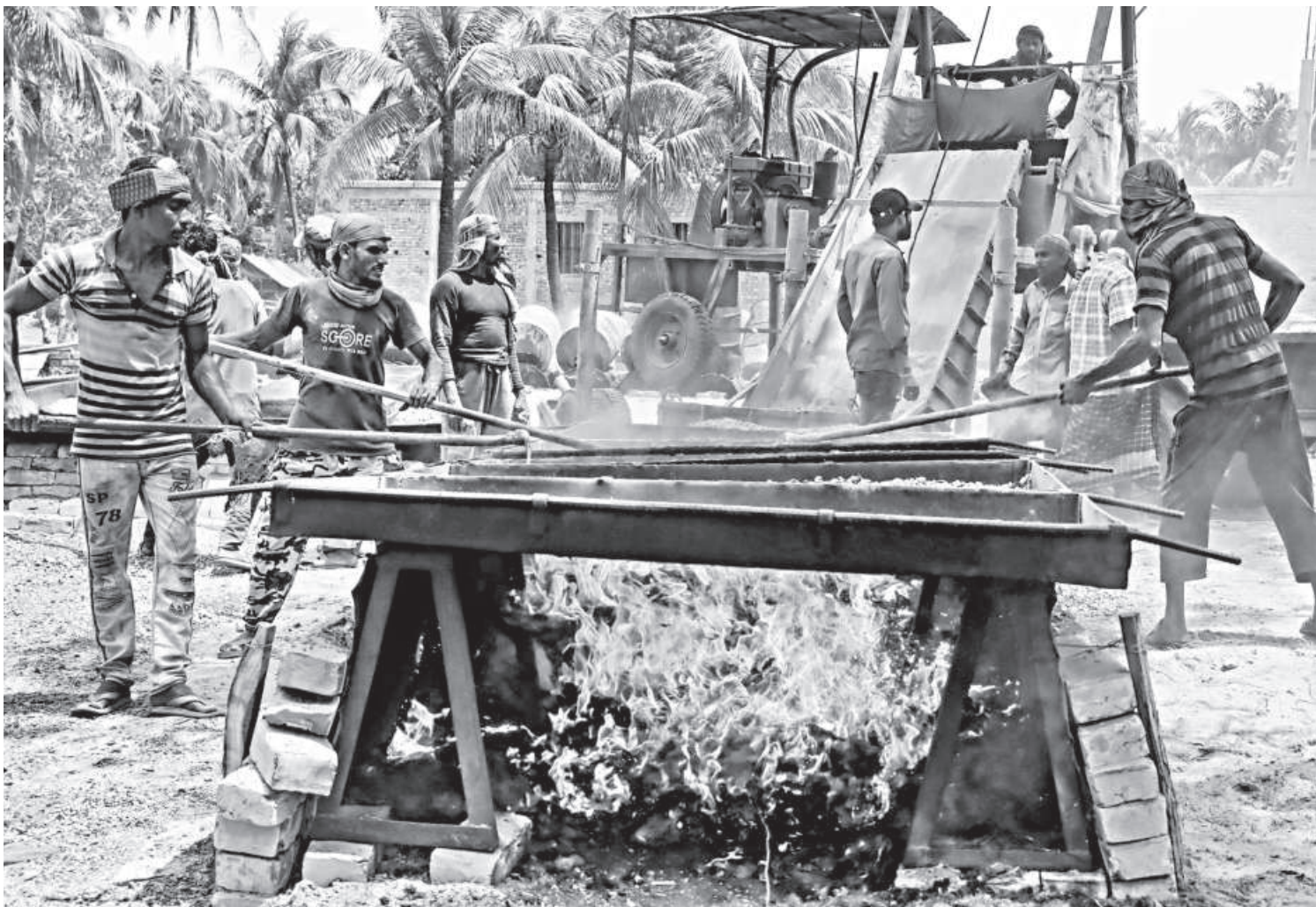
Workers prepare bitumen for roadwork in Khulna. After an entire day of intense labour amid soaring temperatures, they earn around Tk 700. The photo was taken in the Rajbadh area of Batiaghata recently.
