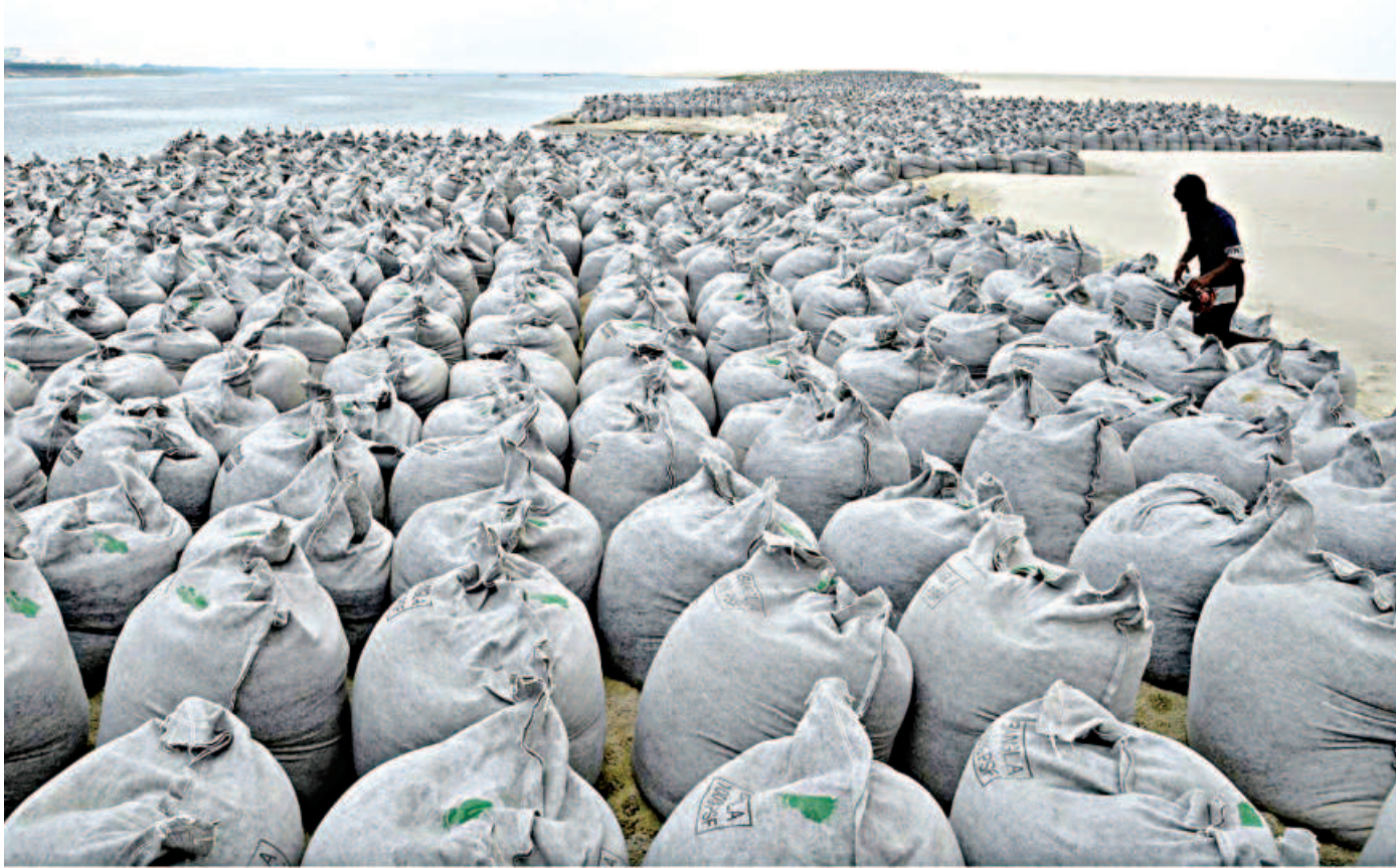
As far as the eye can see, countless neatly arranged sandbags line the bank of the Padma in Rajshahi city. The sandbags are to be dumped into the river as a means to protect the embankment and safeguard the city from potential flooding in the monsoon season. The photo was taken yesterday at the T dam area.
