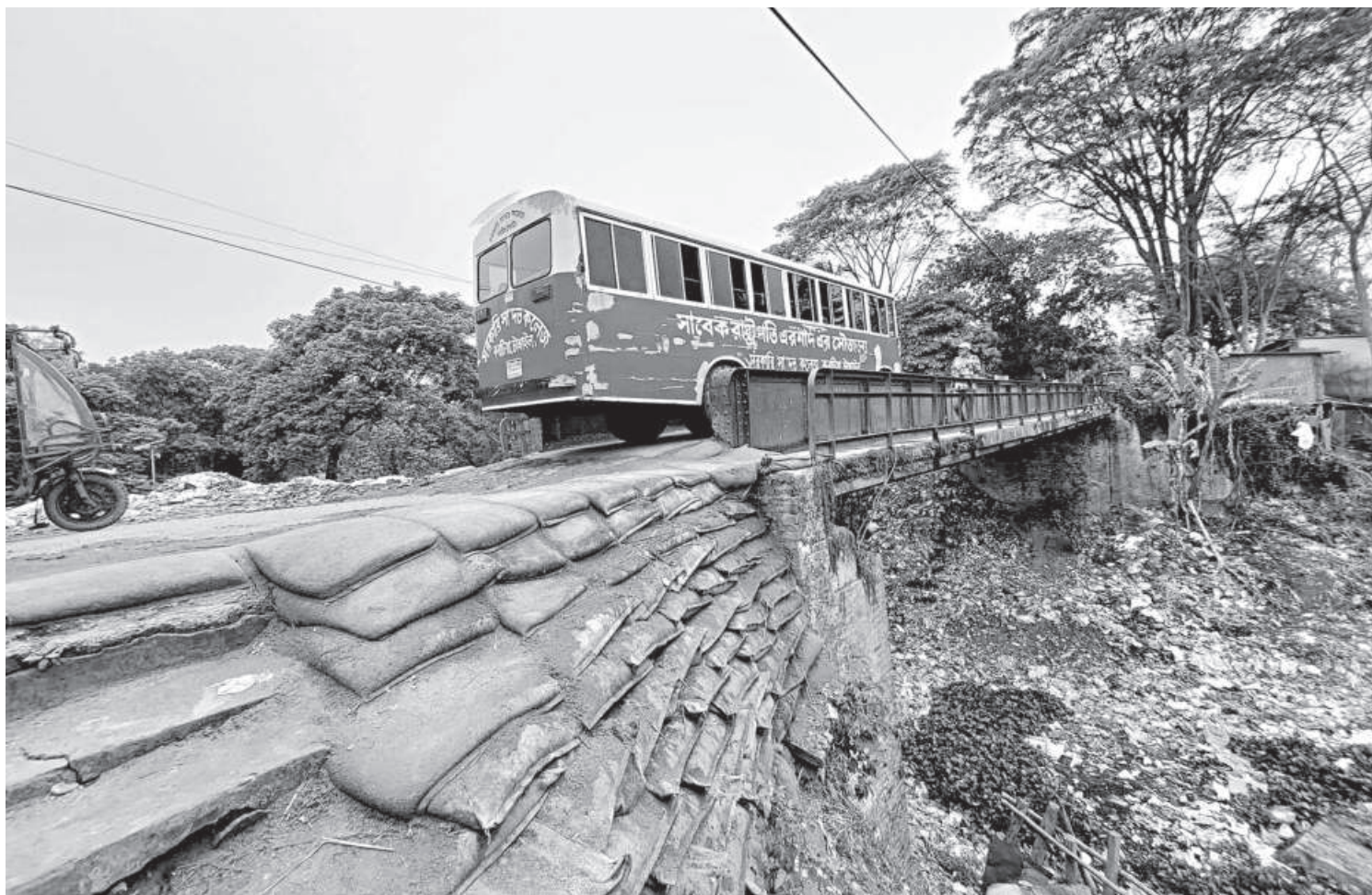
The iron bridge over a canal on the Old Dhaka-Tangail Road lies in a derelict state and could collapse at any moment, leading to a fatal accident. The bridge was constructed around 1952, but has been worn out over the years due to a lack of maintenance and the pressure of hundreds of heavy vehicles crossing it daily. The photo was taken recently.
