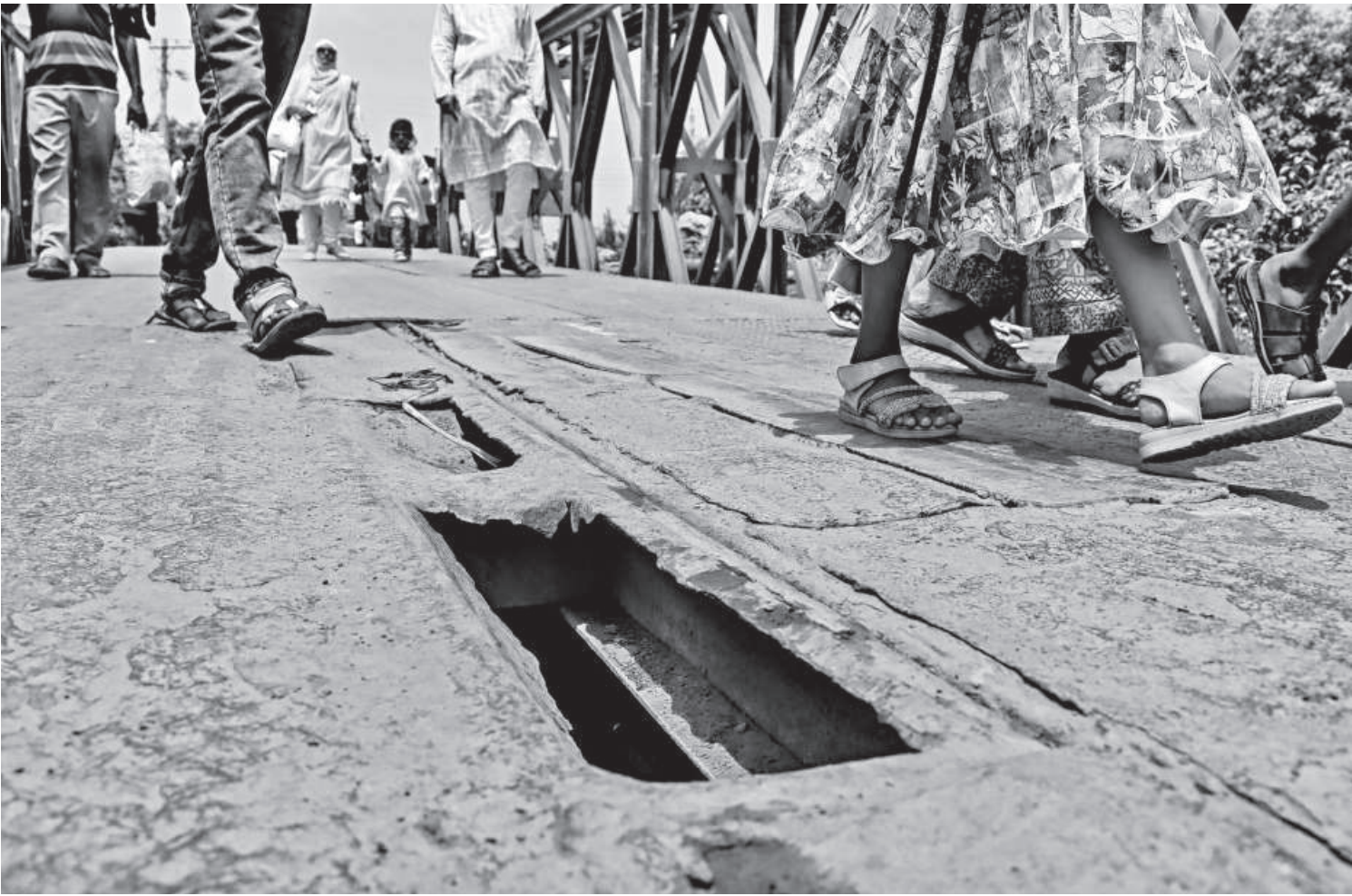
Pedestrians crossing with risk over a broken pontoon at Bagerhat-Mongla ferry terminal yesterday. Over the years, the pontoon has been damaged in various places, causing pedestrians to slip and potentially leading to accidents at any time. Thousands of pedestrians cross the river through this pontoon every day.
