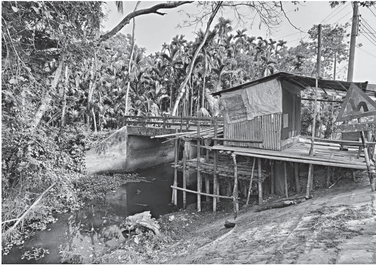
These structures have been illegally built along the Ilisha road in Bhola Sadar encroaching on the canal. Such man-made activities are causing this canal to gradually shrink. The photo was taken yesterday.
