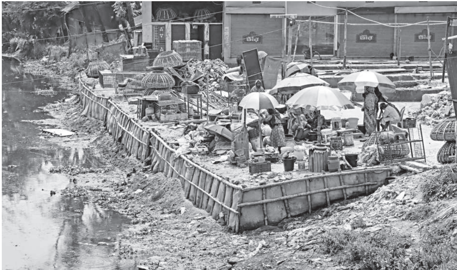
Shops have been set up by filling sand into the river, obstructing the water flow of the vital Mayur River, which was dredged recently. The reduced navigability of the river is now causing waterlogging in various areas of the city during the monsoon. The photo was taken in Khulna's Gallamari area.
