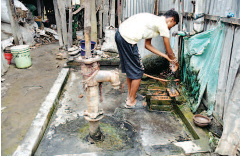
Even though this tubewell is 200 feet deep, the declining groundwater levels prevent it from lifting water during the dry season.
