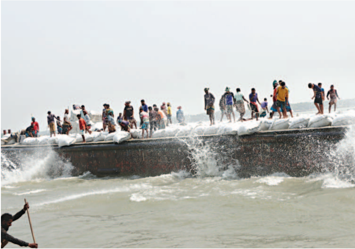
Workers drop geo-bags filled with sand along the banks of the Kirtankhola river in Barishal. In preparation of the upcoming monsoon season, these bags will help prevent erosion at vulnerable points along the riverbank. The photo was taken in the city's DC Ghat area yesterday.
