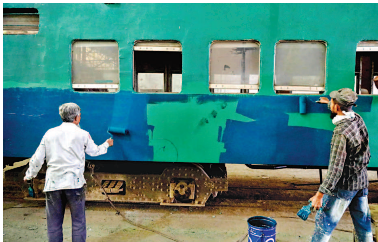
Workers painting a carriage after repairing it at Bangladesh Railway's Pahartoli workshop in Chattogram on Sunday. Work on refurbishing carriages is going on in full swing ahead of the Eid holiday travel rush. The workshop is working on 90 carriages.
