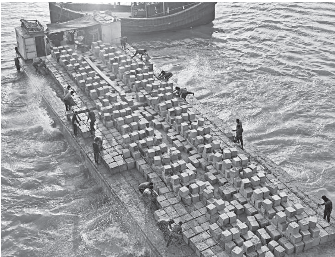
Workers dropping cement, stones, and sand blocks around the pillars of the Captain Mohiuddin Jahangir Bridge (Doarika Bridge). This initiative was taken due to the increased current along the Sugandha River on the Barishal-Dhaka highway. The photo was taken from the Babuganj upazila in Barishal yesterday.
