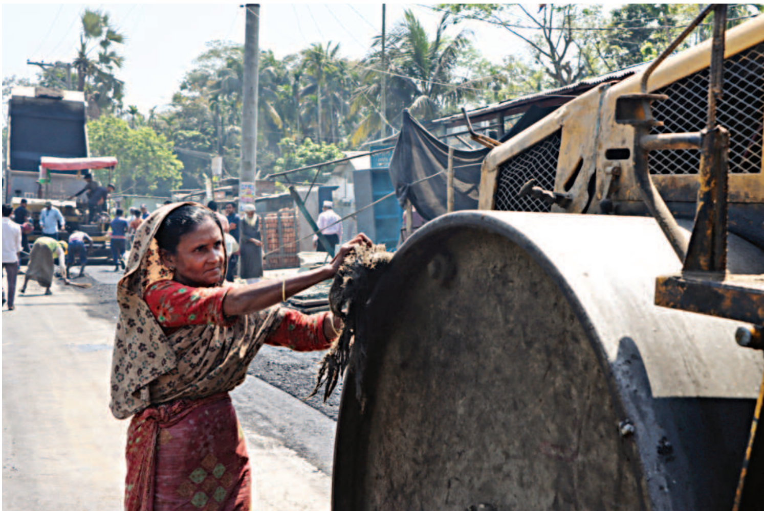
Selina Begum uses a jute sack to spread water and soybean oil to this roller applying bitumen on the Barishal-Dhaka highway. After working from morning to evening, the 56-year-old earns only Tk 500 per day. The photo was taken at Gournadi, Barishal yesterday.
