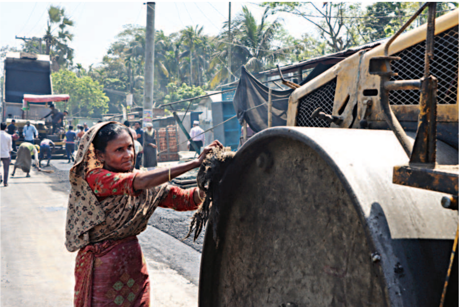
Selina Begum uses a jute sack to apply water and soybean oil to this roller, which is applying bitumen on the Barishal-Dhaka highway. After working from the morning till the evening, Selina earns only Tk 500-600 per day. The photo was taken from the Gouranadi area yesterday.
