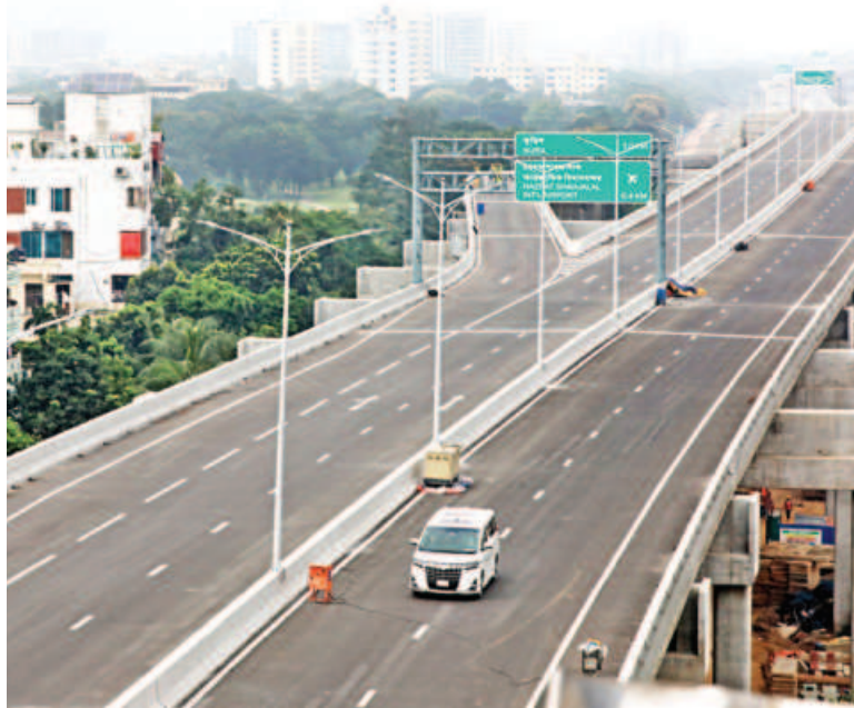
Dhaka Elevated Expressway.
