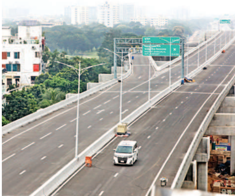
Dhaka Elevated Expressway.
