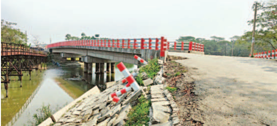
The approach road of this bridge at Uttar Char Montaz village in Patuakhali's Rangabali upazila starts collapsing only a year of its construction.
