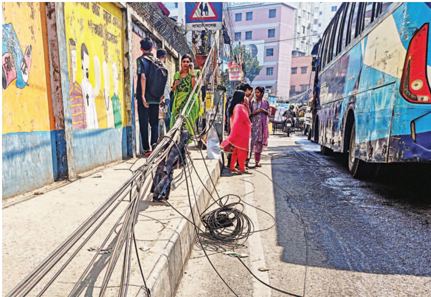
Exposed cables lie across the side of this footpath, posing a risk to pedestrians. The photo was taken in the Bakshi Bazar area yesterday.
