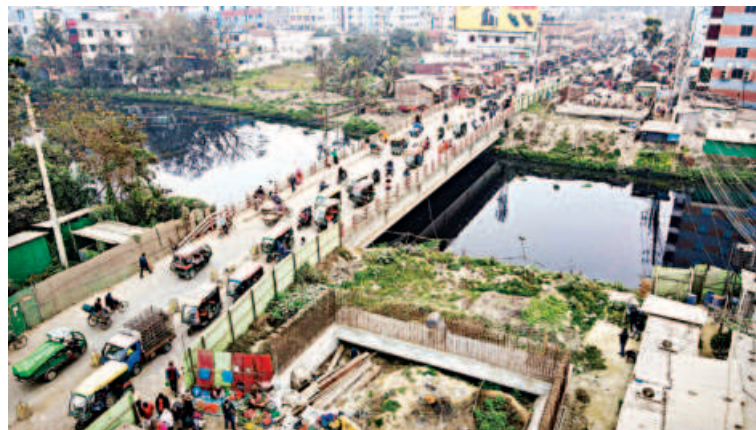
Built too low, Gallamari Bridge, a key gateway to Khulna city, has long been a source of woe for residents due to its faulty design. Meanwhile, the work for a new bridge goes on at a snail's pace, exacerbating public sufferings.
