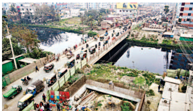
Built too low, Gallamari Bridge, a key gateway to Khulna city, has long been a source of woe for residents due to its faulty design. Meanwhile, the work for a new bridge goes on at a snail's pace, exacerbating public sufferings.
