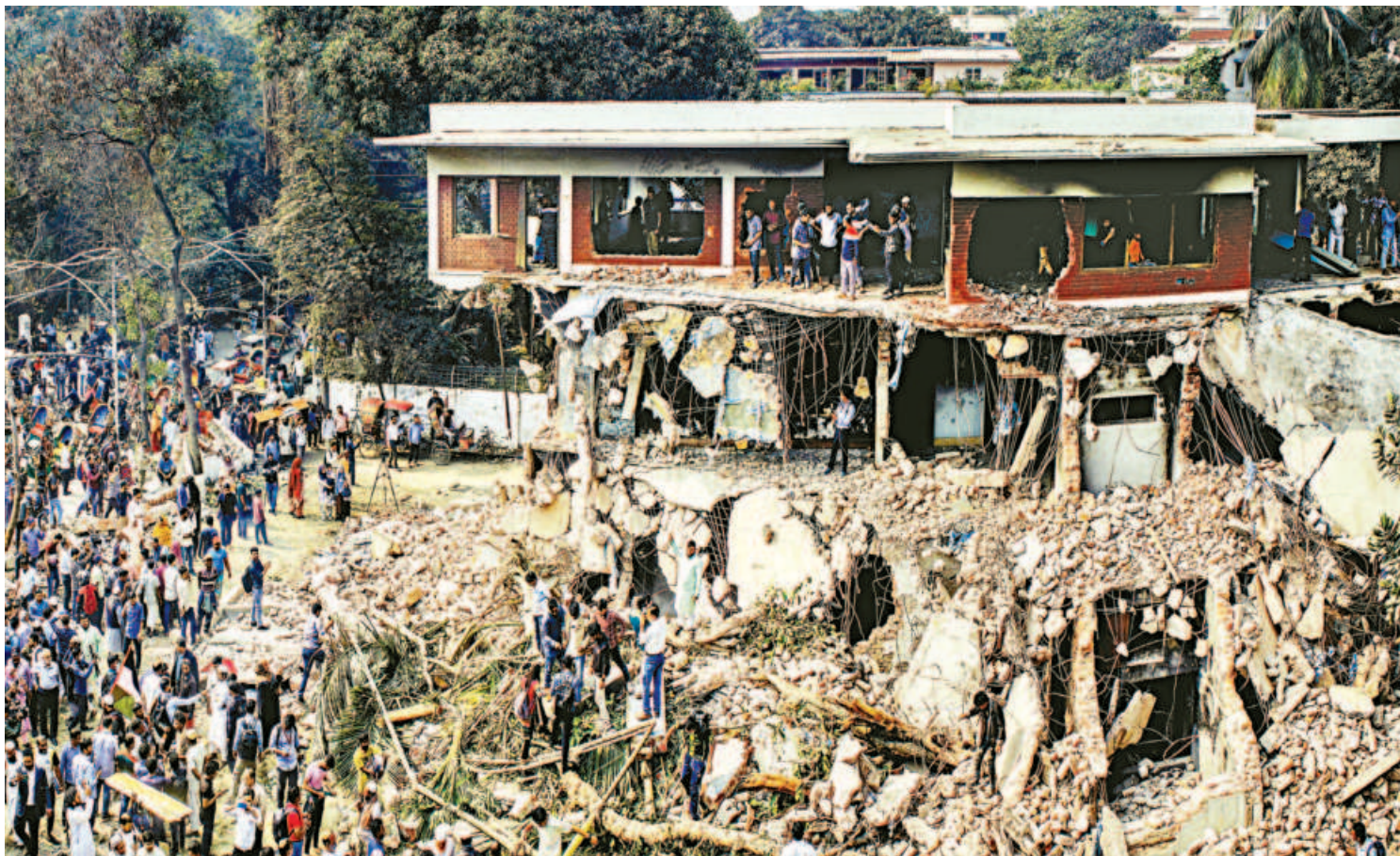
Crowds gathered at Bangabandhu Memorial Museum lying in ruins in Dhanmondi 32 yesterday. The demolition of the building began on Wednesday night and continued till yesterday afternoon.
