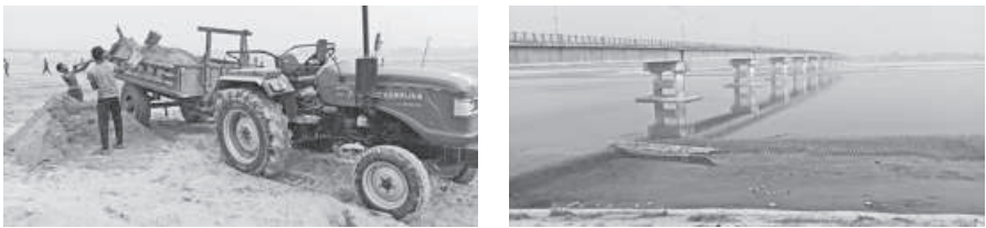
Illegal sand extraction from the Dharla river in Kurigram's Phulbari upazila is posing a threat to the foundations of Dharla Bridge, with the site of the extraction being only 100 metres away from the bridge.
