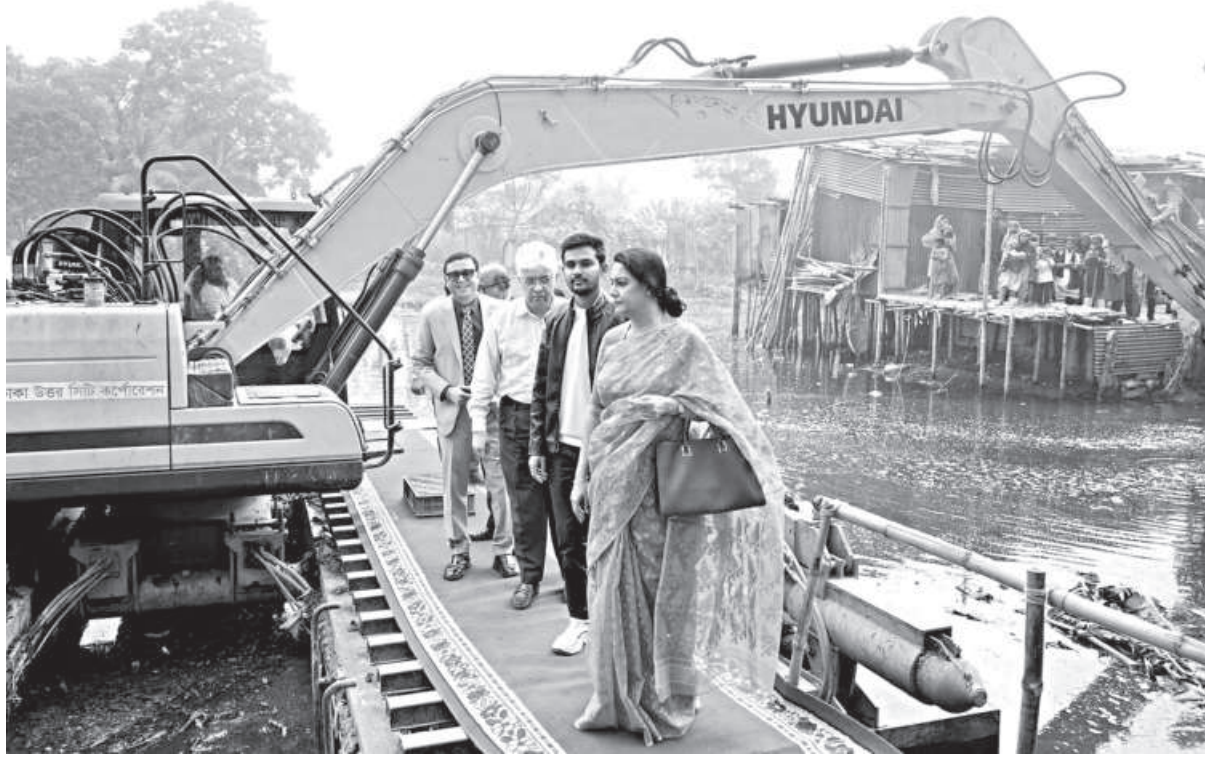
Environment Adviser Syeda Rizwana Hasan; Housing, Public Works, and Industry Adviser Adilur Rahman Khan; and LGRD Adviser Asif Mahmud Sajib Bhuiyan inaugurated the excavation work on six canals yesterday. The photo was taken at the banks of Baunia Canal in the capital's Mirpur.
