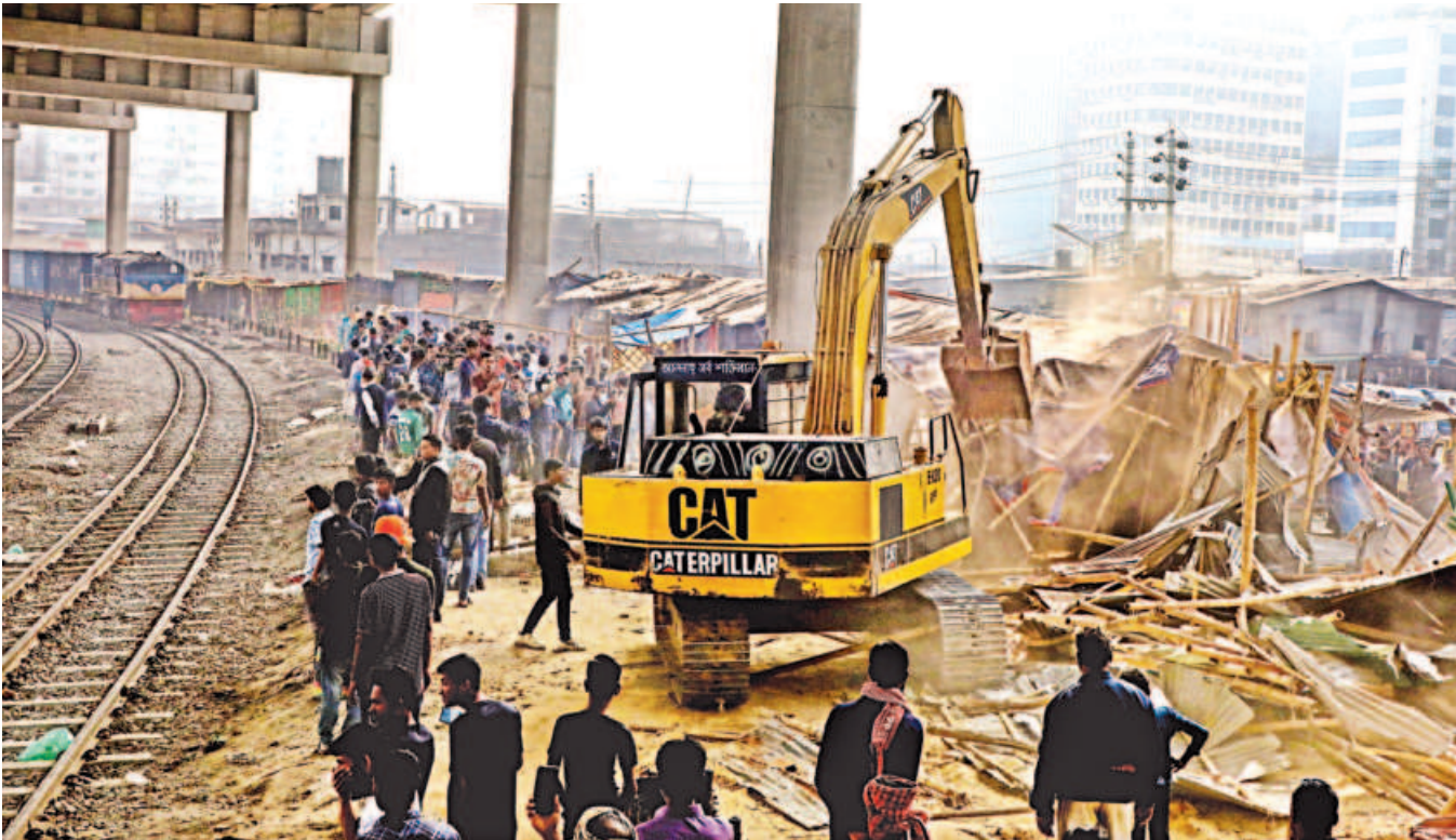
Bangladesh Railway uses a digger to destroy around 100 shanties built on its land at Karwan Bazar in the capital during an eviction drive yesterday. PHOTO: PRABIR DAS
