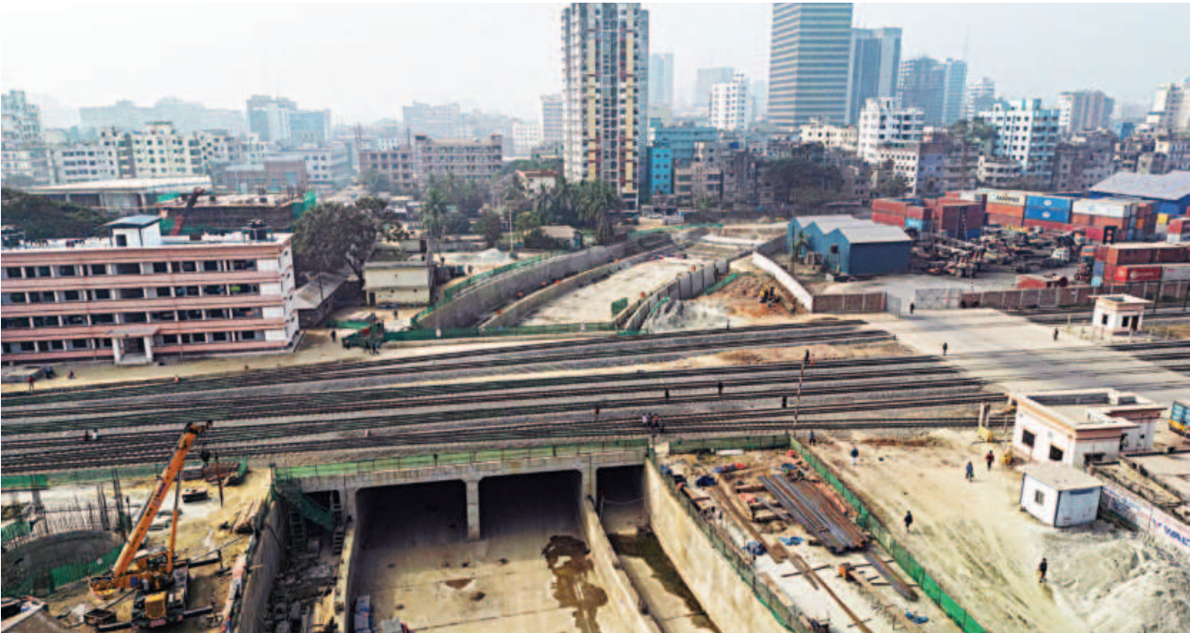
This photo of a construction site at Titipara, Kamalapur, shows the six-lane underpass project, which is being implemented at a cost of around Tk 100 crore. Upon completion, this infrastructure will allow vehicles to navigate smoothly via the underpass while trains can run uninterrupted on the railway lines above.
