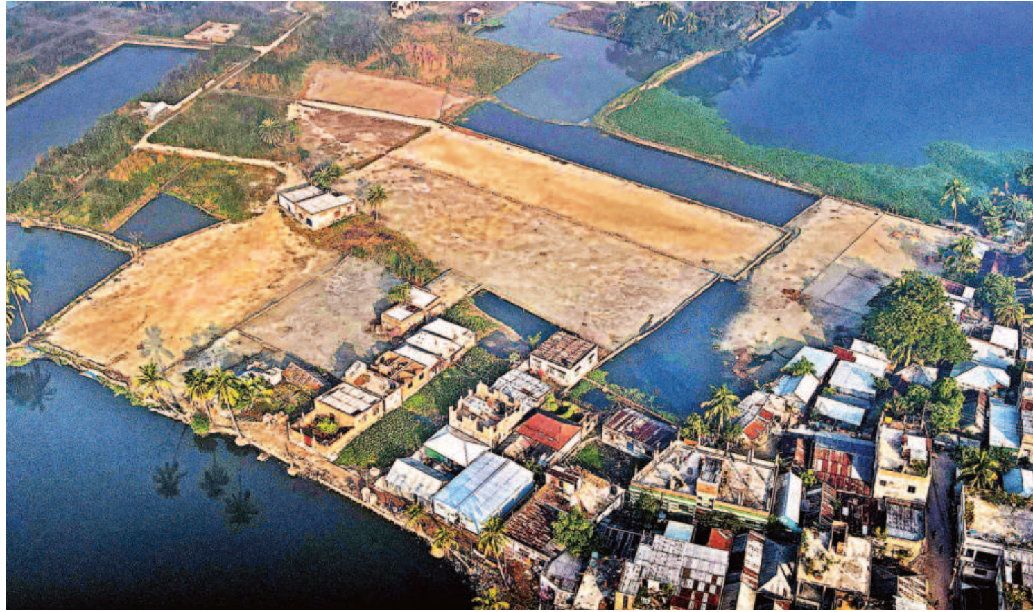
A large swathe of wetland in Khulna city's Khalishpur has been filled with sand to make way for a housing project. This has not only hampered the biodiversity but also increased the chances of flooding in the area. Such unplanned housing projects are largely behind the shrinking of agriculture lands and wetlands. The photo was taken recently.
