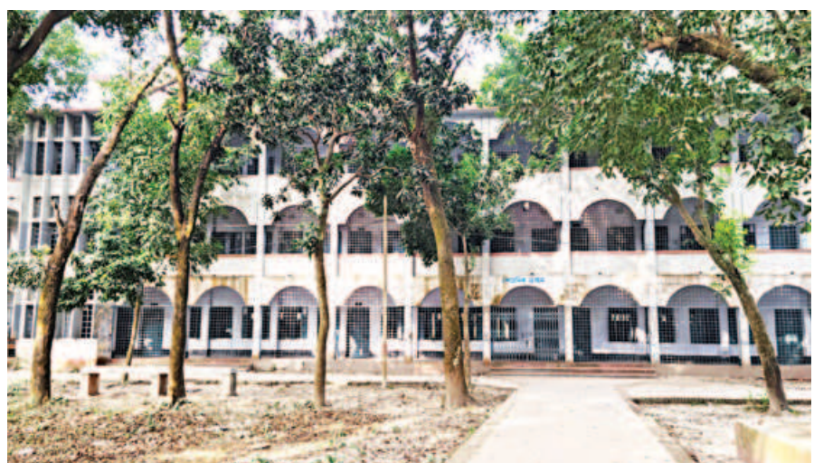
The old academic building of Phulbari Government College in Dinajpur's Phulbari upazila.
