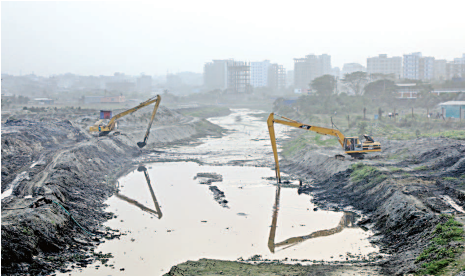
Workers dredging a canal using excavators near the Madani Avenue area yesterday. Under the supervision of Bangladesh Water Development Board, work is ongoing to restore navigability of this waterbody. Constant dumping of waste and poor management over the years have left many canals in the capital in such a sorry state.
