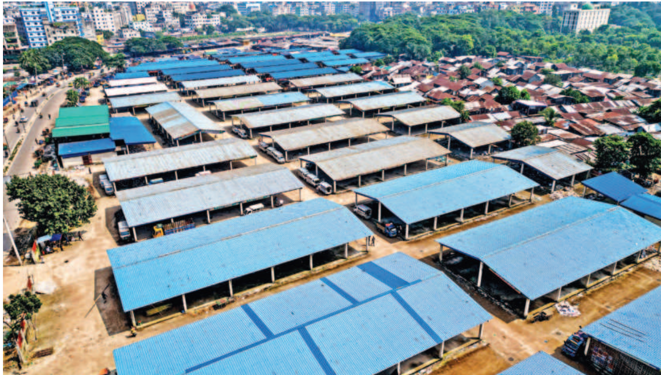
Mirpur Diabari Agricultural Product Market remains mostly empty since its construction in 2019 as traders say the market is located far from the city centre, while there are other markets in the area. Locals allege the empty sheds are often used for criminal activities. This photo was taken recently.
