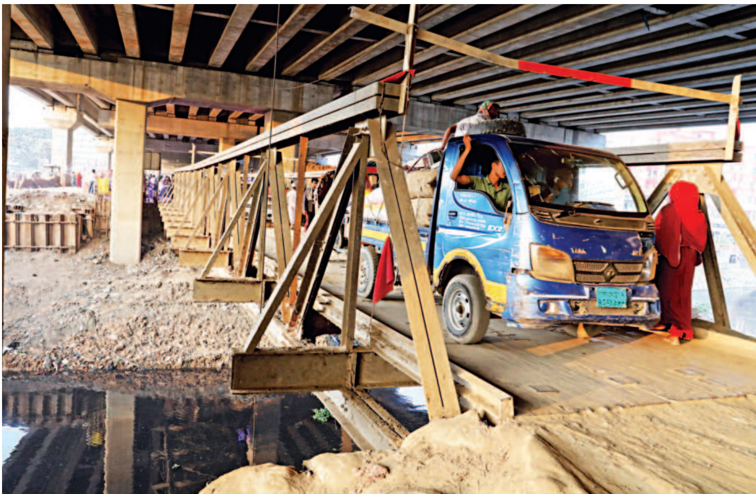
A goods-laden pickup crosses a rickety bailey bridge over the Turag river beneath a flyover in Tongi, Gazipur. Although the bridge is designed only for lighter vehicles, it is frequently used by the heavy ones. This practice led to the collapse of a nearby bailey bridge last week, yet drivers continue to use this one amid risk. The photo was taken at Abdullahpur recently.
