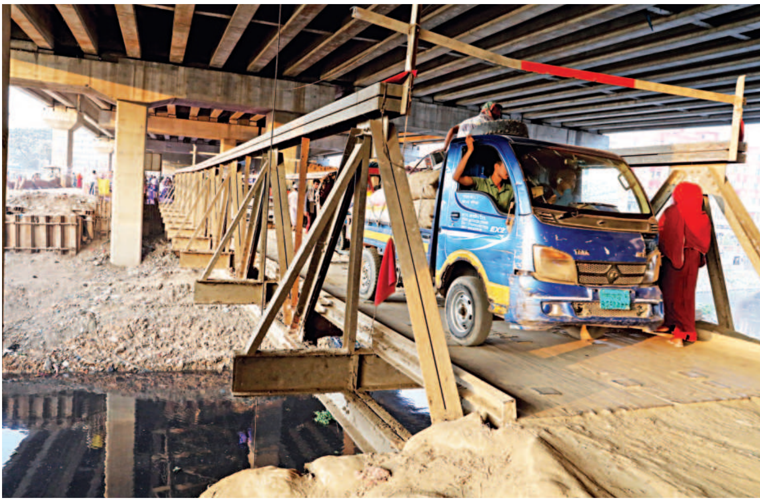
A goods-laden pickup crosses a rickety Bailey bridge over the Turag river beneath a flyover in Tongi, Gazipur. Although the bridge is designed only for lighter vehicles, it is frequently used by the heavy ones. This practice led to the collapse of a nearby Bailey bridge last week, yet drivers continue to use this one amid risk. The photo was taken at Abdullahpur recently.
