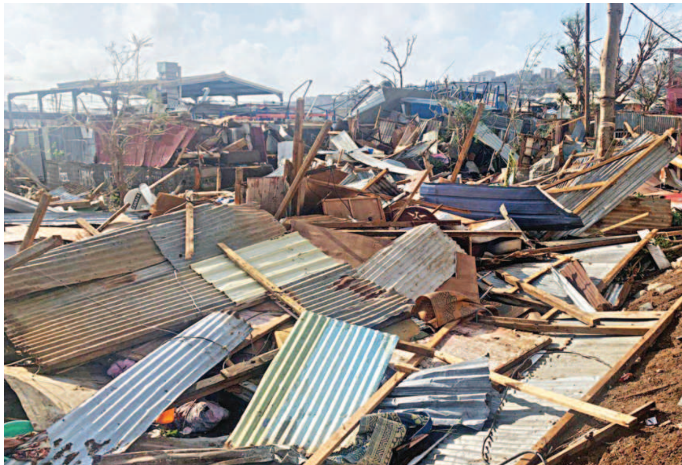
This handout photograph, taken on Sunday and released yesterday, shows a pile of debris of metal sheets and wood after the Cyclone Chido hit France's Indian Ocean territory of Mayotte.
