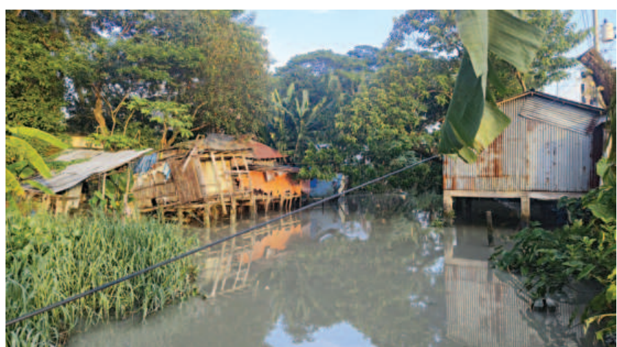
A section of local people have continued encroachment on Basugi Khal in Barguna's Amtali upazila. PHOTO: STAR
