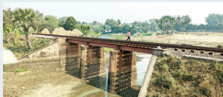
Present photo of Sahagola Bridge in Atrai upazila, Naogaon. Part of the bridge was demolished during an operation on Sept 6, 1971. An incoming Pakistani train was derailed, and over 100 enemy soldiers were killed in a subsequent gunfight.
