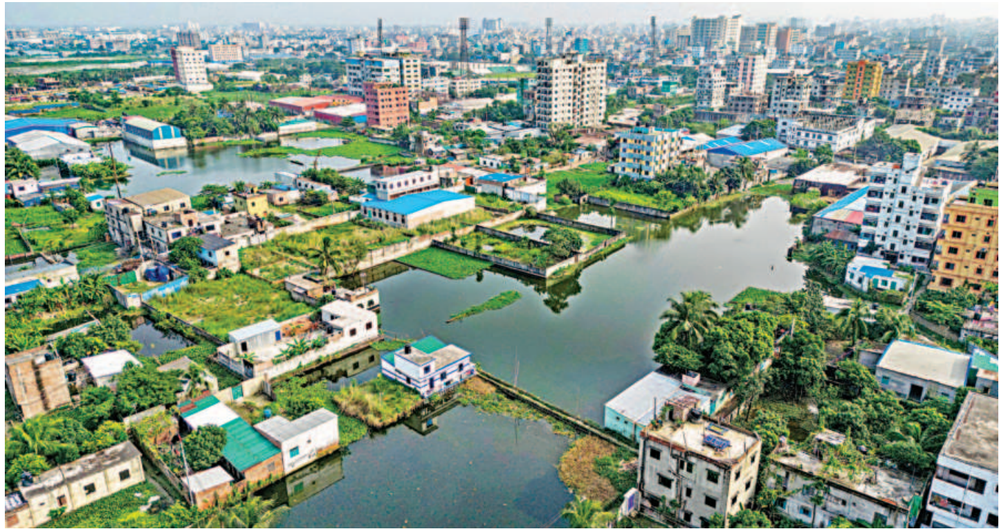
Unplanned and unregulated development of residential and factory buildings in the low-lying area of Fatulla, Narayanganj, has caused waterlogging. Many of the buildings can only be accessed via bamboo bridges. The area, which lacks proper drainage, remains flooded almost throughout the year, and the stagnant water gets polluted. The photo was taken recently.
